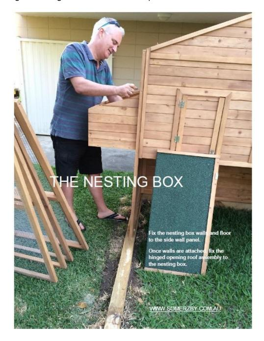
Fix the nesting box walls and floor to the side wall panel.
