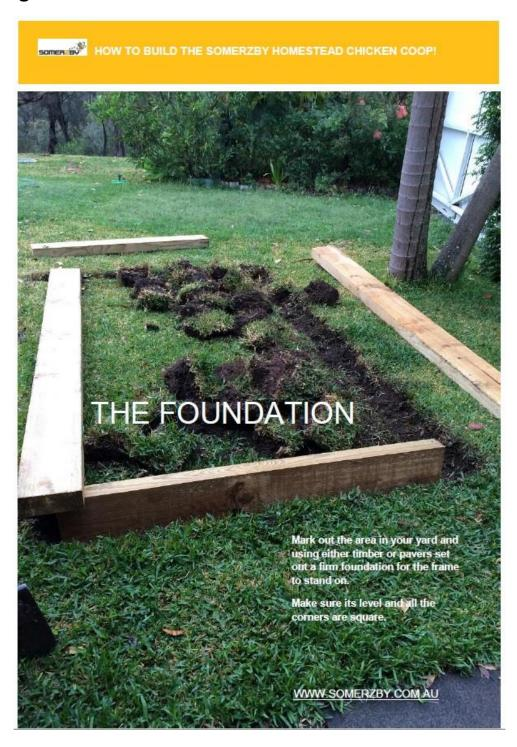
Mark out the area in your yard and using either timber or pavers set out a firm foundation for the frame to stand on.
