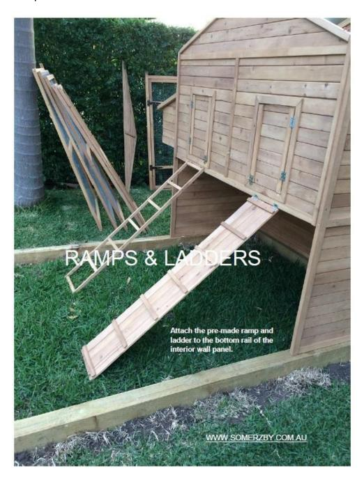
Attach the pre-made ramp and ladder to the bottom rail of the interior wall panel.
