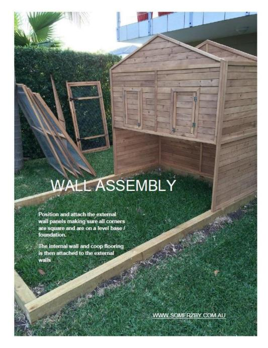
Position and attach the external wall panels making sure all corners are square and are on a level base / foundation.
