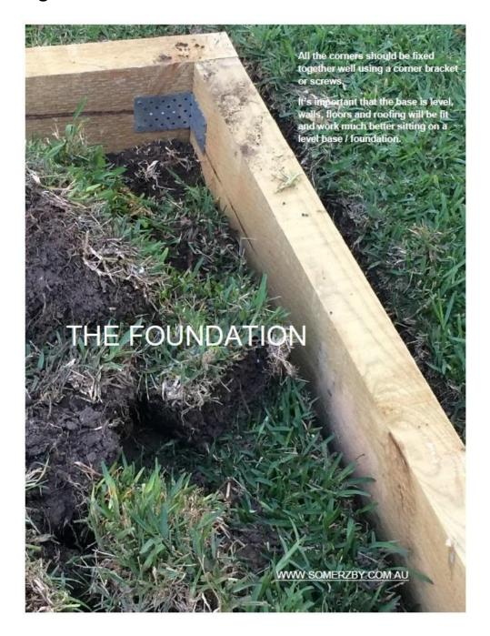
All the corners should be fixed together well using a corner bracket or screws.
